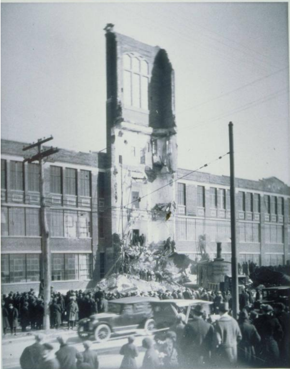
Title Fuller Brush building following collapse of tower, 1080 Windsor Avenue, Hartford
