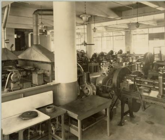
ROLLING MILL - HEAT TREAT AND PRESS AREA
