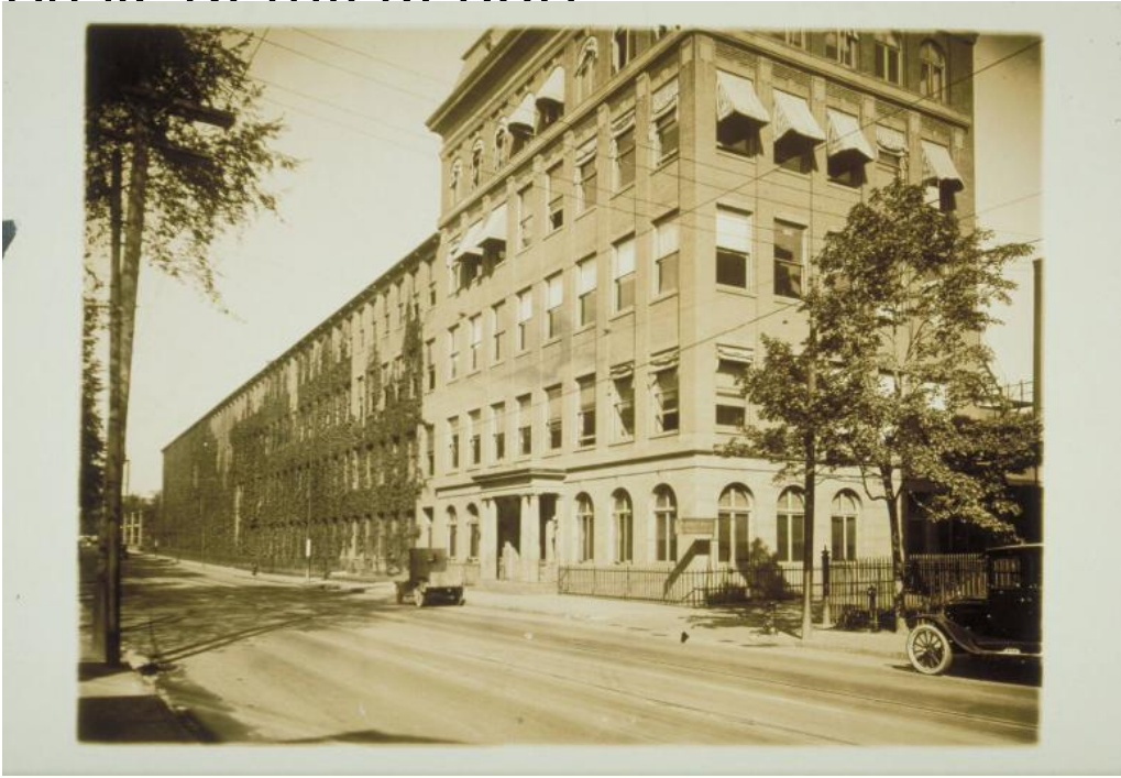
Title Hartford Machine Screw Co.: exterior of factory building, Capitol Avenue, Hartford
