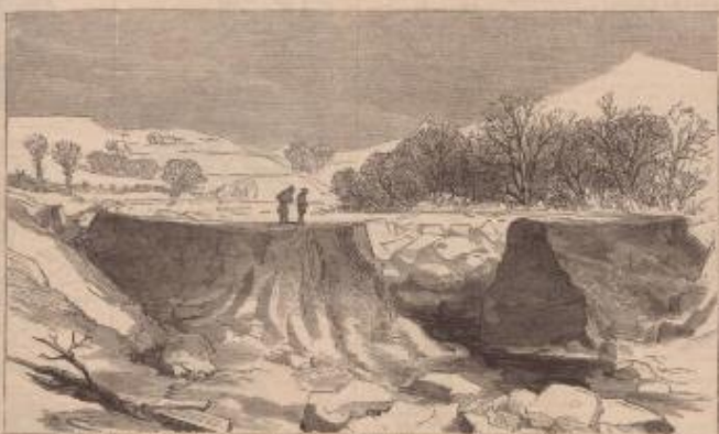
TERRIBLE DESTRUCTION AT BANGOR, MINNESOTA, JANUARY 21, 1888.—RUIN OF THE CYRUS DAM.—(Features on THE S. D. DAM.)
