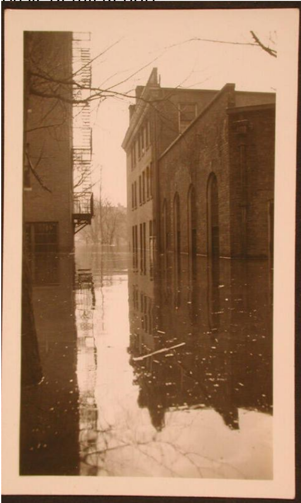
Title Flood Waters Between Buildings, Hartford
